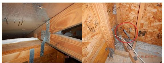
**Type of Roof to Wall Connectors**: Standard Metal Straps/ Good condition at accessible areas of the Attic- I observed one strap in the Garage Attic at the South Wall that is not fastened to the Wood Frame Wall/ We recommend having a qualified contractor evaluate the loose Strap and properly secure it at the Frame and Wall
