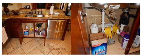
Kitchen Sink- Previous leak stains were noted at the left side Kitchen Sink but no active leaks were present at the time of the Home Inspection/ This location should be monitored over time for reemergence of previous leaking condition
