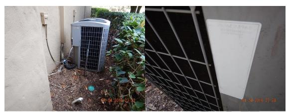
Two of the Condenser Units are installed at the north side of the building/ These are for the Master Bedroom and the First Floor Main Living Area Systems
