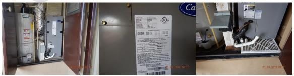
Air Handler Unit installed at the Second Story Exterior Closet at the West Balcony for Master Bedroom System
