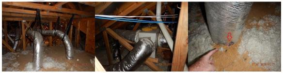
Ducts visible at the Second Story Attic- Minor repair recommended for damaged Duct close to the Attic Access Panel
