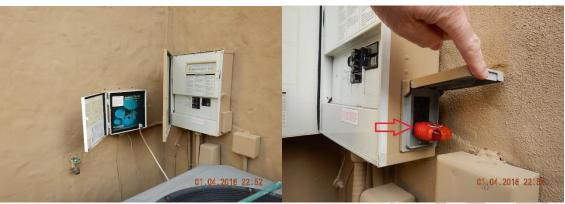
GFCI Receptacle is not tripping when tested at the Pool Panel
