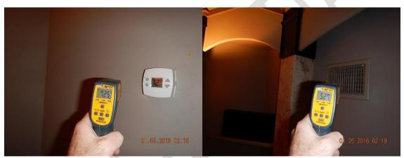
Movie Room System produced cool air when operated during the Home Inspection/ One of the vents in the Movie Room is connected to the 5 Ton Second Floor System
