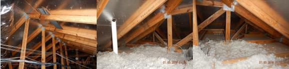
**Type of sheathing**: 15/32" Plywood/ **Condition**: Good condition at visible & accessible materials- Radiant Heat Barrier inhibited viewing access to the majority of the Roof Deck Materials
