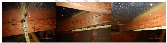
Roof Decking Attachment Nail Size & Spacing: 8d nails spaced a maximum of 6" apart in the field/ I used a Metal Detector to locate and estimate the nails and calculate the spacing
