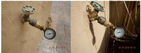
Overall water pressure: 70 PSI- Leak at the Hose Bib at the South Exterior Wall should be repaired at the Pool Area-The Hose Bib leaks at the handle when under pressure
