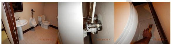
Movie Room Hallway Bathroom Areas- Reset loose Toilet and Wax Ring/ Active moisture was detected with a Moisture Meter at the Bathroom Floor close to the Toilet which could indicate possible leaking from the Wax Ring at this time
