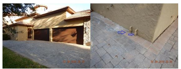
Main Shut off Valve #1 & # 2 Location: South Exterior Wall-Southeast Corner at the Laundry Room- Repair or replace (2) Main Water Shut off Valves located at the South Exterior Laundry Room Wall/ The Valves do not fully turn off the water into the home
