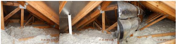
Attic Insulation: R- 30 Loose Fill Fiberglass-Fiberglass Batt-Radiant Heat Barrier/Good condition and evenly installed throughout accessible areas of the Attic
