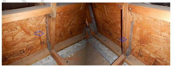
Type of Roof to Wall Connectors: Standard Metal Straps/ Good condition at accessible areas of the Attic
