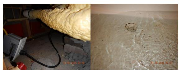
There is dirt in the Tub Jet System and the Air Blower function appears compromised at this time/ The Service Access Panel is installed the left side of the Tub/ GFCI Protection was verified
