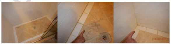
Further evaluate cracks in the Tiles at the Shower and Wall Tiles in the East Second Floor Hallway Bedroom Bathroom/ The cracked tiles may allow water to penetrate and rust the Shower Pan over time
