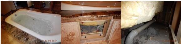
The Jacuzzi Tub in the Master Bathroom was filled and operated during the Home Inspection/ The Tub is functional but requires further evaluation at this time/ There is dirt in the Tub Jet System and the Air Blower function appears compromised at this time/ The Service Access Panel is installed the left side of the Tub/ GFCI Protection was verified
