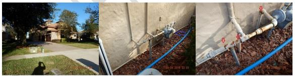
Rust at Gas Lines at the South Exterior Wall
