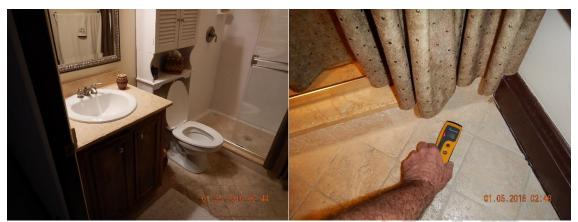
Further evaluate cracks in the Tiles at the Shower and Wall Tiles in the East Second Floor Hallway Bedroom Bathroom/ The cracked tiles may allow water to penetrate and rust the Shower Pan over time/ Active moisture was detected with a Moisture Meter at the time of the Home Inspection at the Bathroom Floor which could be an indication of a problem at the Shower Area at this time
