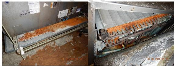
5 Ton Air Handler Unit should be serviced at this time/ Rust was observed in the overflow pan and typical mold stains were observed at the Air Handler Cabinet Areas
