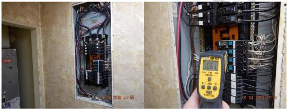
Visible and accessible wiring appeared to be in good condition at the time of the Home Inspection- Infrared Thermometer indicated elevated temperatures at the AFCI Breakers
