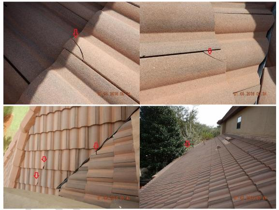
There are several Tiles with minor cracks that were observed at several areas at the Roof and some areas where mortar has cracked. The Roof is dues for standard maintenance at this time to repair minor chips and cracks and also to repair minor separation at mortar areas at the Roof Ridge areas
