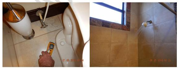
Second Floor Hallway Bathroom Areas- Reset loose Toilet and Wax Ring at the Second Floor Hallway Bathroom/ Active moisture was detected with a Moisture Meter at the Bathroom Floor close to the Toilet which could indicate possible leaking from the Wax Ring at this time
