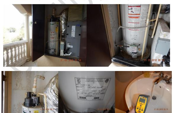
The Water Heater at the Second Floor West Balcony Closet appeared functional and in good condition/ The Water Heater was replaced in 2012 and produced hot water during the Home Inspection
