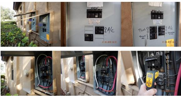
The Main Service Disconnect Panels are installed at the South Exterior Wall/ Both Panels and visible and accessible wiring appeared to be in good condition at the time of the Home Inspection
