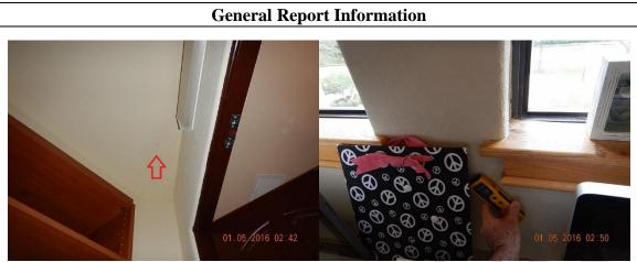
Evidence where previous moisture may have been present in the Bedroom Closet at the East Hall Bedroom and at the bottom left corner of the window in the Second Floor Study were tested with a Moisture Meter and found dry at the time of the Home Inspection indicating the areas have not been recently wet
