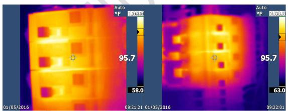
This prompted me to take Infrared Photos of the Panel which also illustrated the AFCI Breakers were running hot
